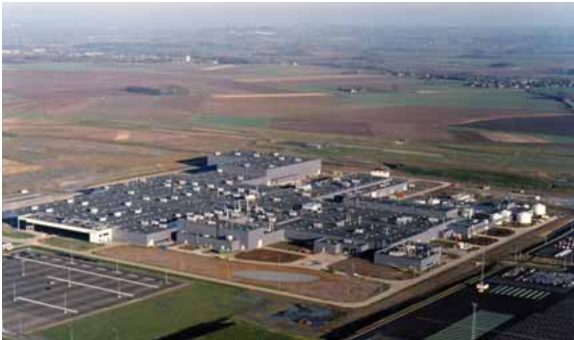
Toyota’s manufacturing plant in Valenciennes, France.
